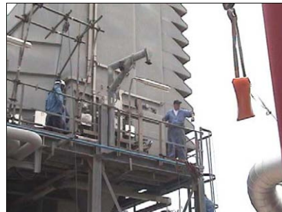
Figure 13: Skid in use with crane
